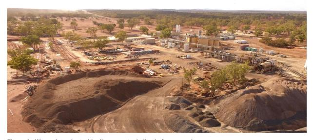
Figure 2. Wonawinta plant with silver ore stockpiles in foreground
