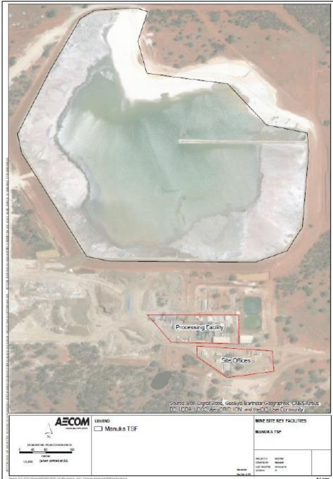
Figure 3 – Key Site Facilities Downstream of Manuka TSF
