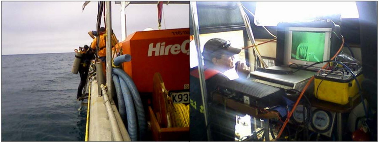
Figure 3-2: Drilling is Diver Operated and Monitored from the Boat
