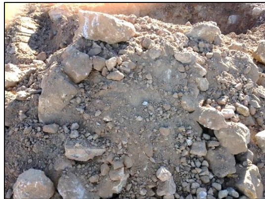
Photograph 8. Excavated material at the Limestone Low Grade Stockpile.
