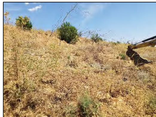
Photograph 20. View of batter on the TSF with vegetation growing directly in the Waste Rock Oxide materials (Site WROR2). Groundcover was 80–100 %.
