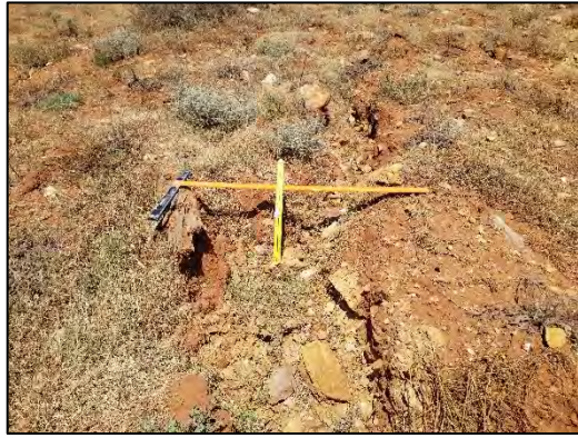
Photograph 21. Rill at Site WRE Rehab 1. Depth approximately 0.25 m, width is 0.15 - 0.5 m.
