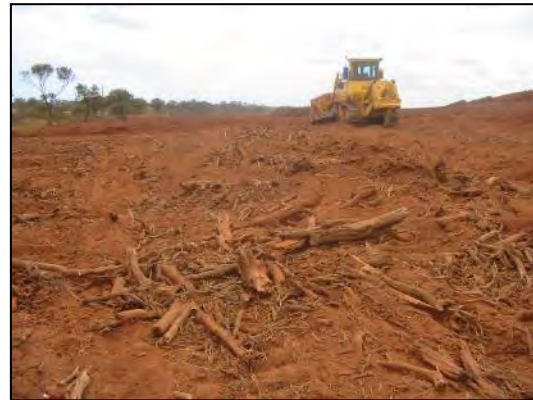
Photograph 25. Spreading tree debris on freshly placed topsoil - Murrin Murrin Operation, WA.
