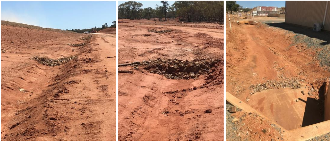
Figures 10 a) and b) TSF run off drain repairs and c) Stormwater drain re-establishment around Plant
