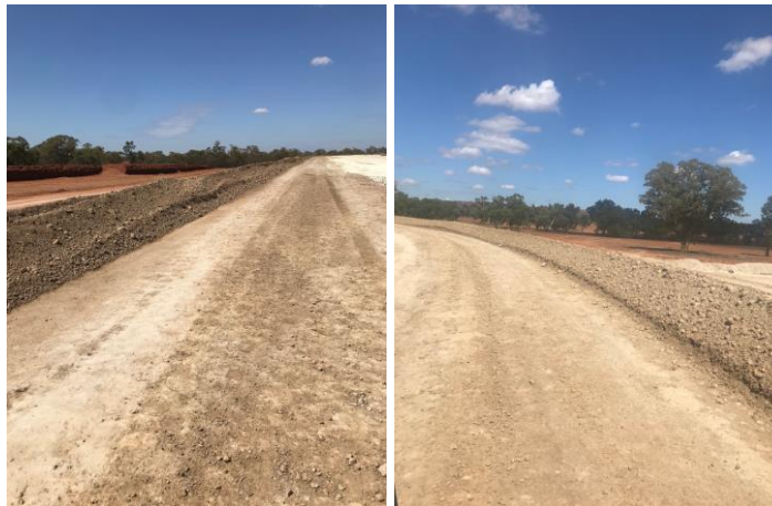
Figures 10 d) and e) TSF windrow repairs
