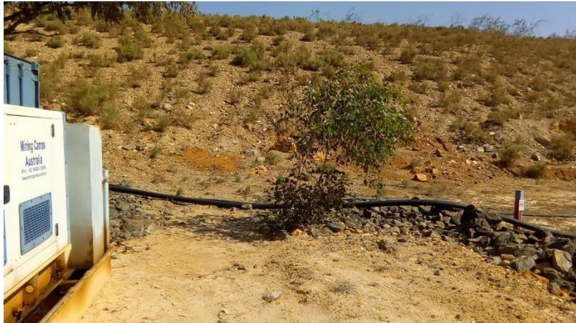
Figure 5: **Northern side of TSF embankment with established groundcover, representing the target groundcover levels.** Photo taken February 2019.
