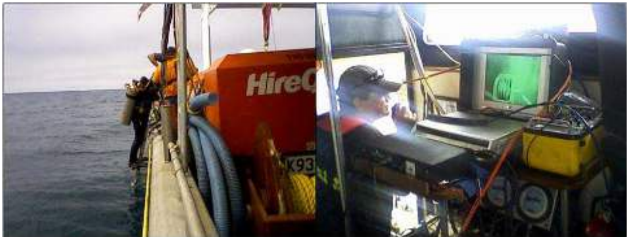
Figure 4-15 Drilling is Diver Operated and Monitored from the Boat
