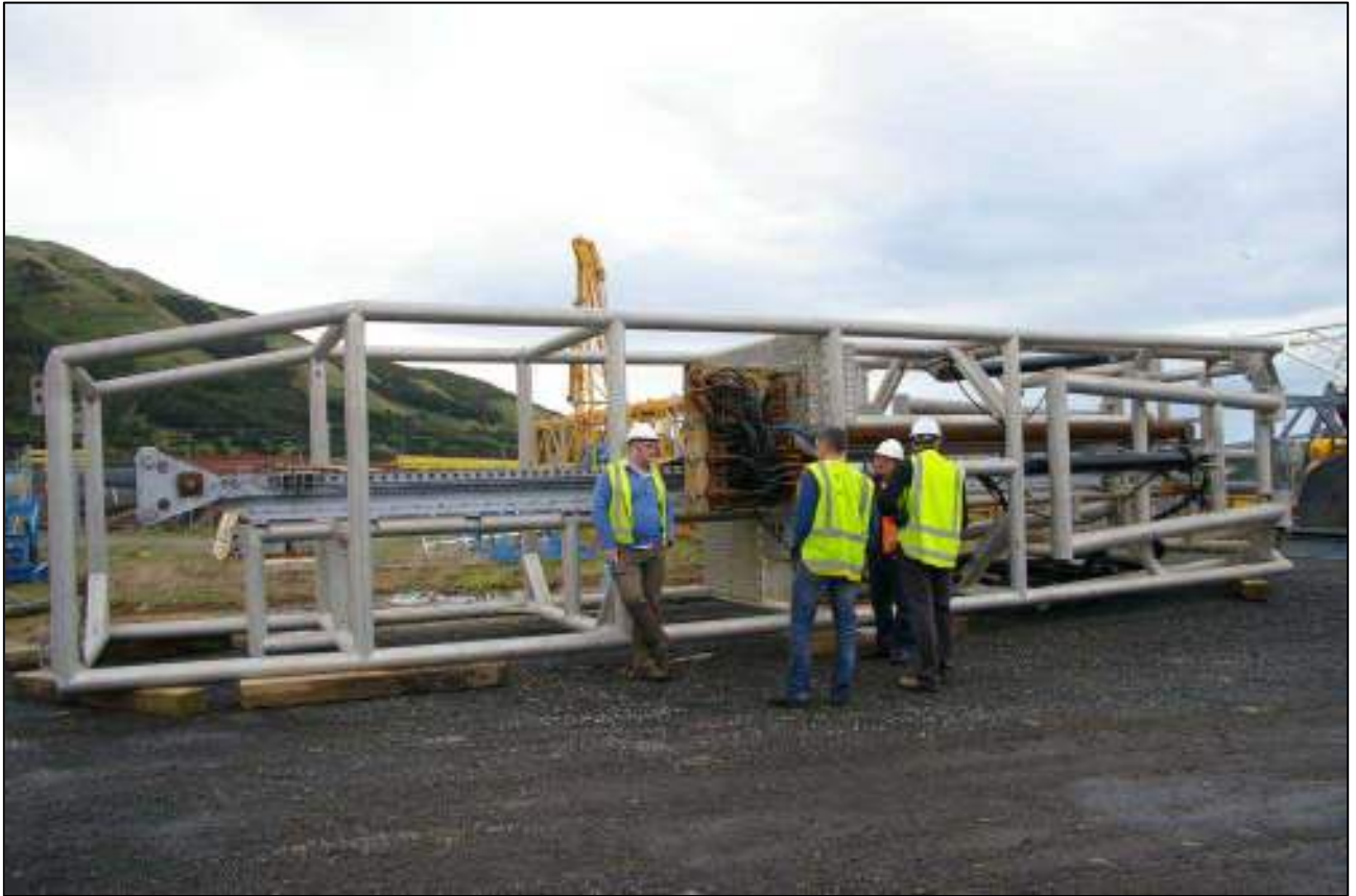
Figure 4-17 Deep Drill Rig TTR Yard Porirua
